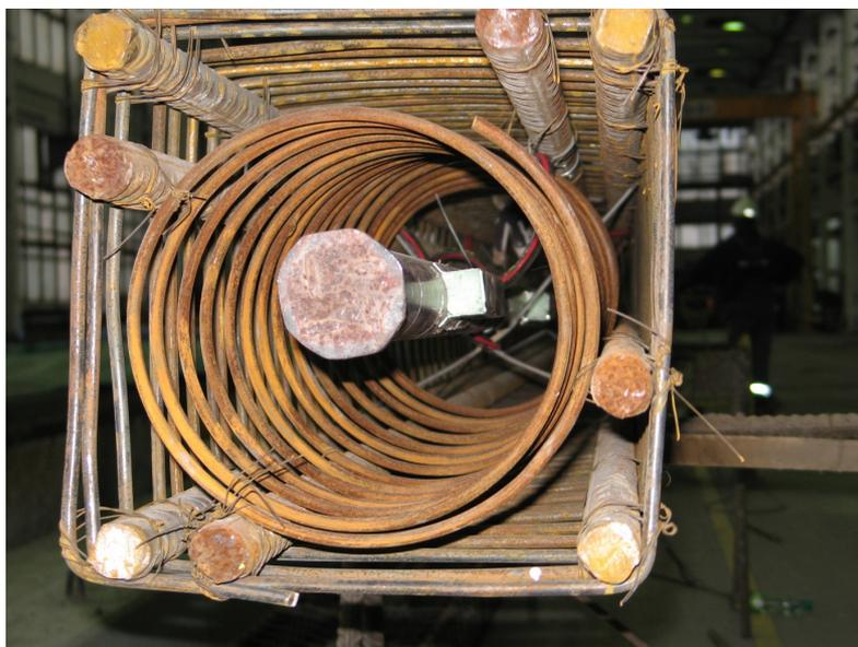
*Fig. 2 Reinforcement cage of a pile T8 with the instrumentation*
