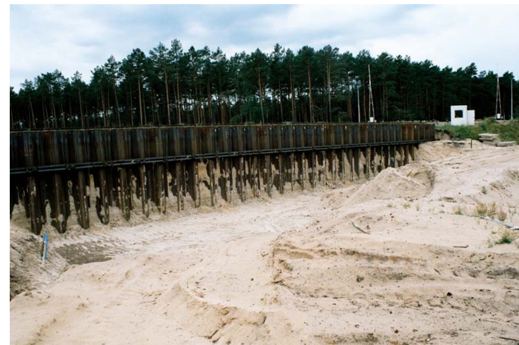
Fig. 1 View of the sheet-pile wall at the support P2.
